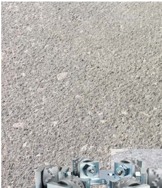
Profile of concrete after one pass with the HTC Ravager™
